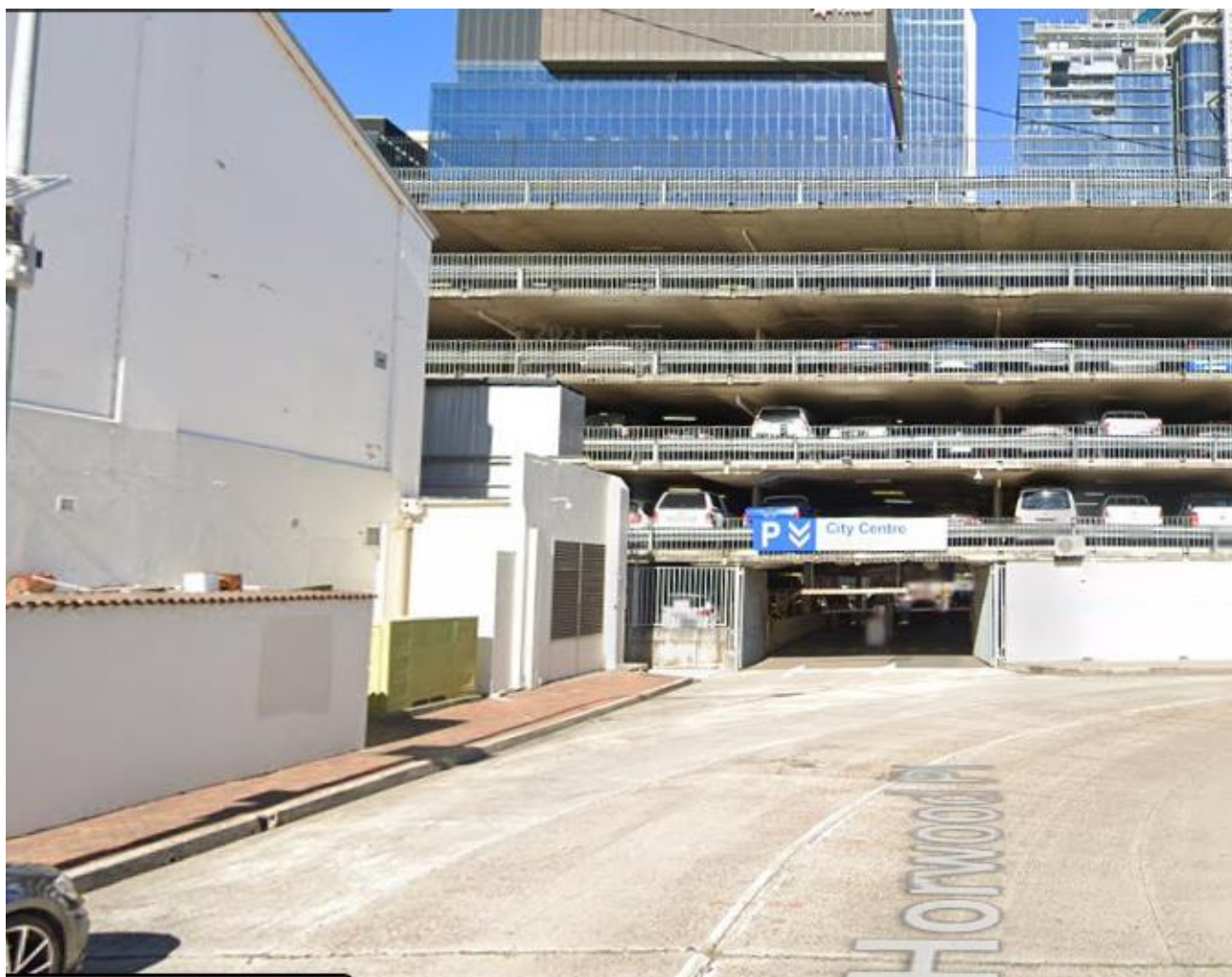
Figure 9: City Centre car park
