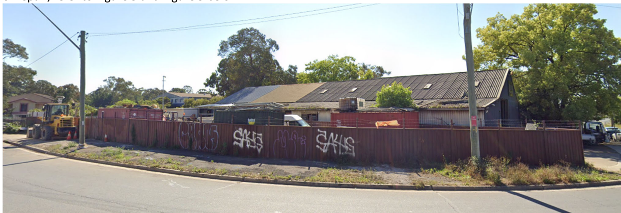
Figure 9: Kay Street/ Unwin Street footpath
