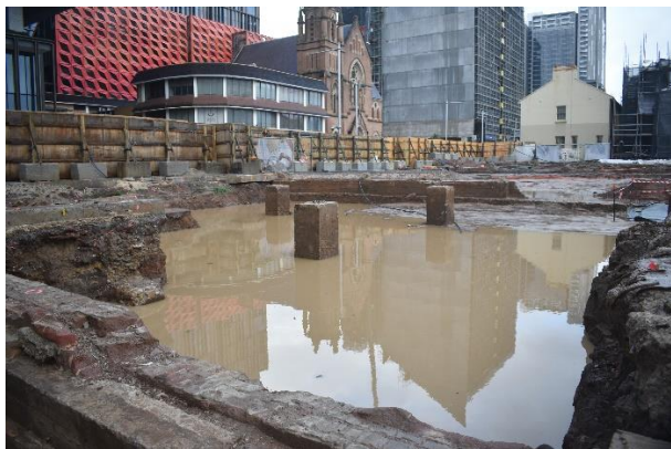
Figure 3.2 Area A, Lot 75, under water following heavy rains in July 2022. Photograph taken looking southwest, towards Macquarie Street.
