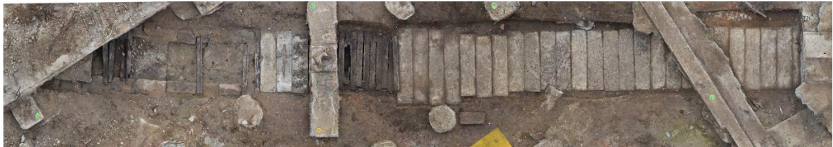
Figure 4.11 Orthophotograph of the Town Drain showing the timber and concrete capping. Several concrete beams were erected to support the 1950s office buildings. (Source: Guy Hazell for GML)
