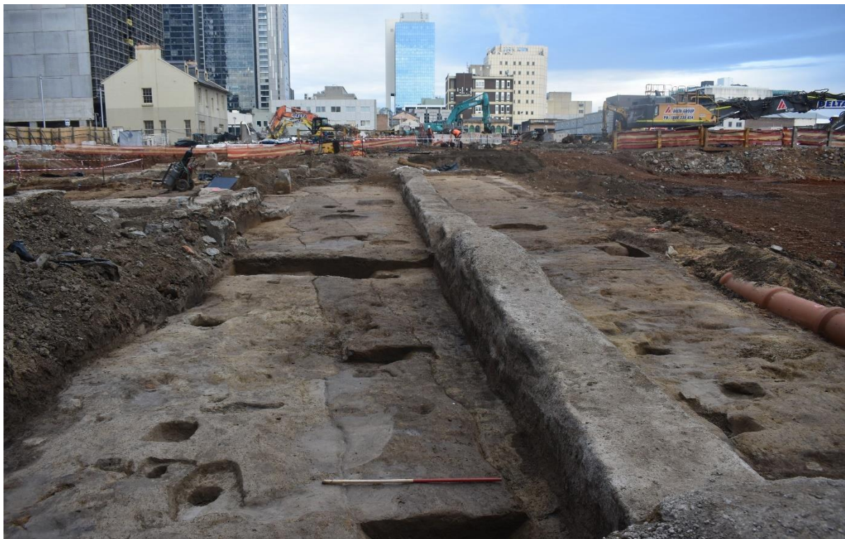
Figure 4.2 A long linear drainage ditch through Lots 76, 75 and 74 dates to the 1790s–1800s and is associated with early cultivation activity prior to development from the 1810s. Photograph is taken looking west. Scale is 1m.
