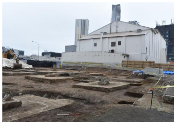
Figure 1.4 Archaeological excavation under way behind the Roxy within Area B and the station box excavation footprint. This area contained large pad footings from the multilevel carpark. Photograph taken looking north.
