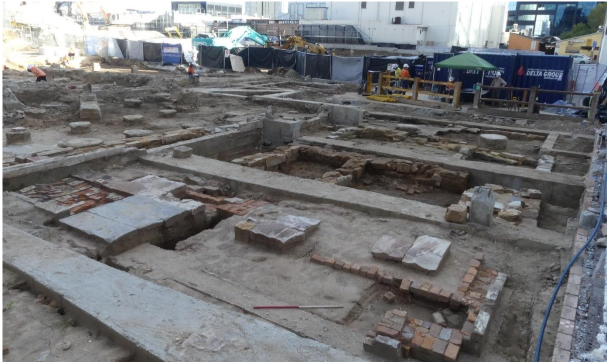
Figure 4.13 The sandstone footings of the substantial two-storey brick house built by the 1850s in Lot 74. The front verandah comprised brick footings and sandstone paving. The archaeology was impacted by concrete footings, piles and beams of the two-storey office building developed on the lot in the 1970s. Photograph taken looking northwest. Scale is 1m.
