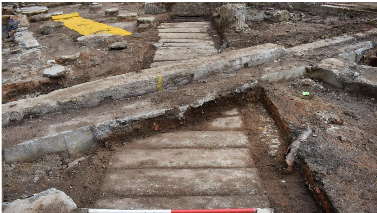
Figure 4.12 The portion of the Town Drain recovered during archaeological investigations of Lot 74. It shows the early twentieth-century concrete covers and substantial mid-twentieth century concrete beams over the drain. The photograph is taken looking southwest towards Macquarie Street. Scale is 1m.
