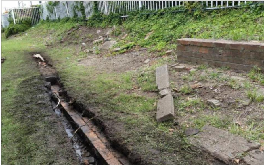
Plate 5: Platform at Hamilton Station classified as a 'work' by the project archaeologist, Wickham Transport Interchange project, 2015
