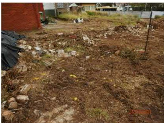
**Photo 9:** Ground surface south-west of 29 Alexandra Avenue - fibre cement debris unexpected finds marked with yellow paint.
