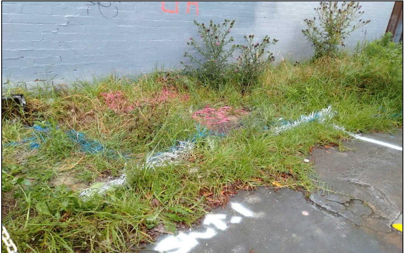
**Photograph 5:** service locating prior to intrusive works, observed at test pit 4. Date: 12.11.21
