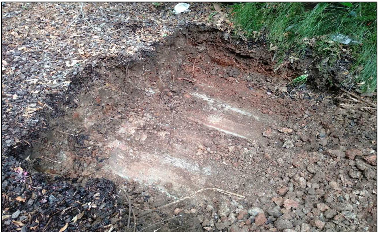
**Photograph 16:** Unexpected buried concrete slab, encountered at TP19. Date: 23.11.21.
