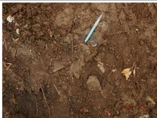
**Photo 10:** Ground surface north of 33 Bailey Street following rainfall event – asbestos debris visible after soil has been washed off surface.
