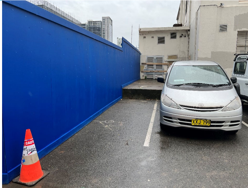
Figure 2: Hoarding installed through car park space
